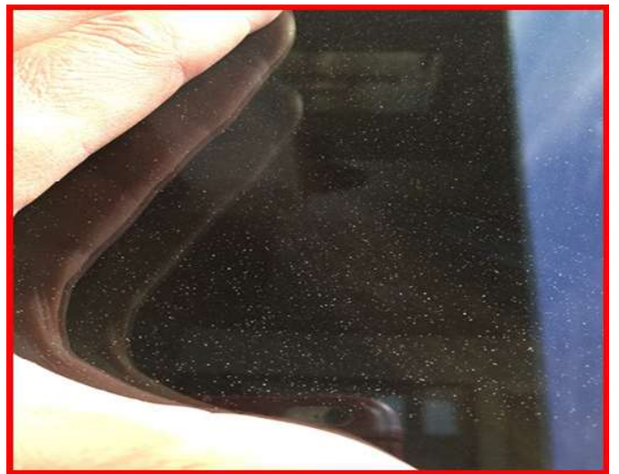
Photo 17-120(4): Paint overspray on multiple windows
